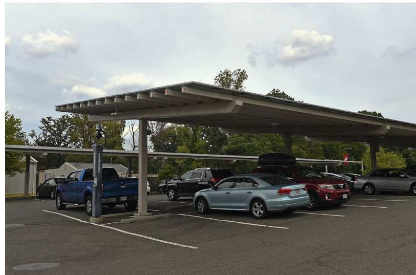
Solar canopy at O'Boyle Parking Lot
